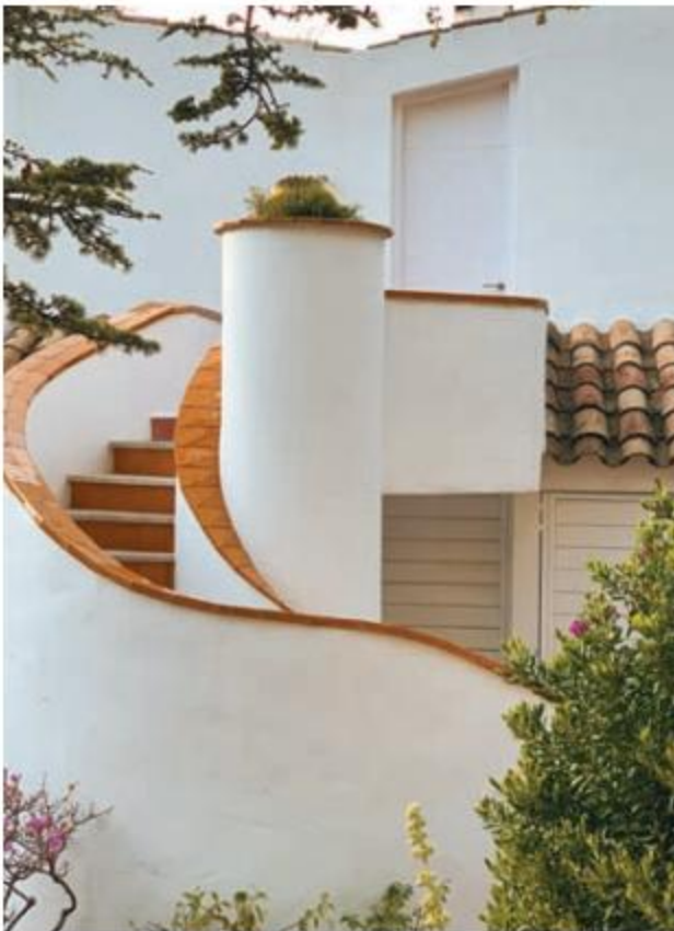
Outdoor application of tile, Spain
